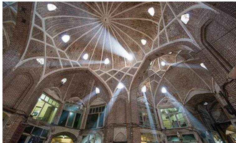
Picture 4. Creation of local lights in different directions in the market of Tabriz and the change of light and shade during the days and seasons.
